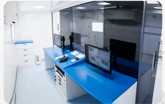
Sala de control Control room
